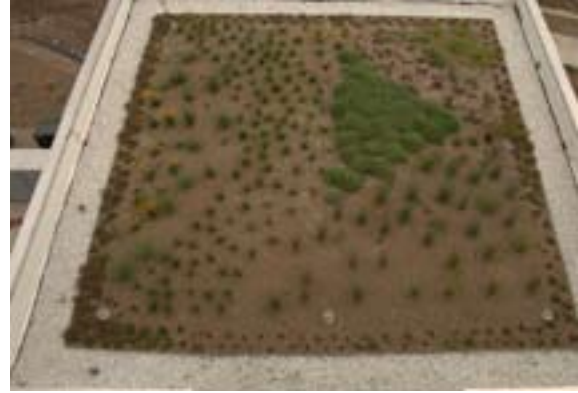
Portions of the new roof is green. Green roofs keep the building cooler, absorb rainfall and reduce storm-water runoff.
